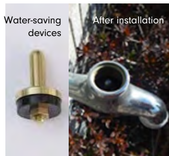
Installation of water-saving devices.
