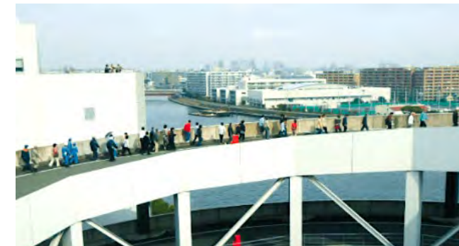
Slope supports people evacuating to the roof top
