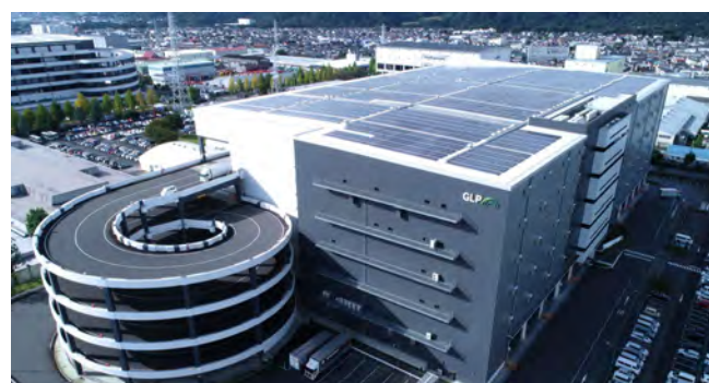
Evacuation base & distribution hub for relief goods
