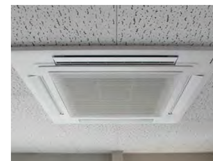
Updating air-conditioning equipment
