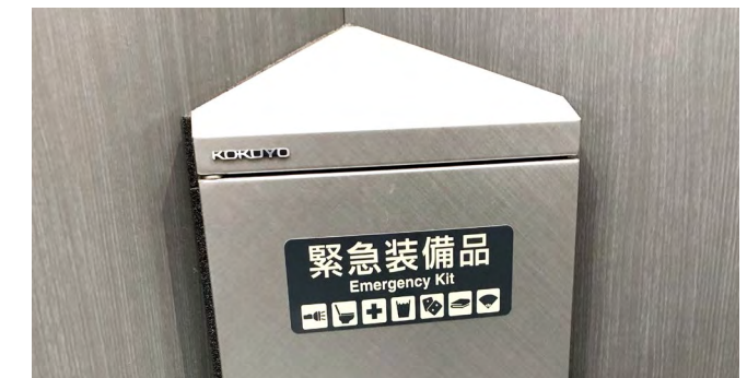
Installing in-elevator fire prevention cabinets
