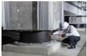
Seismic isolation structure
