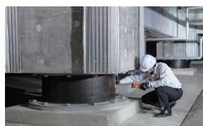
Seismic isolation structure
