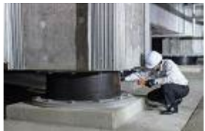
Seismic isolation structure
