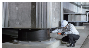
Seismic isolation structure
