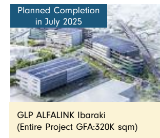
Planned Completion in July 2025 GLP ALFALINK Ibaraki (Entire Project GFA:320K sqm)
