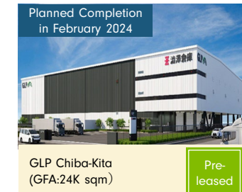
Planned Completion in February 2024 GLP Chiba-Kita (GFA:24K sqm) Pre-leased
