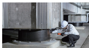
Seismic isolation structure
