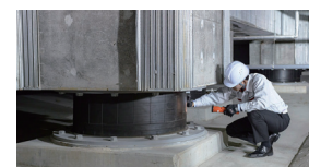
Seismic isolation structure
