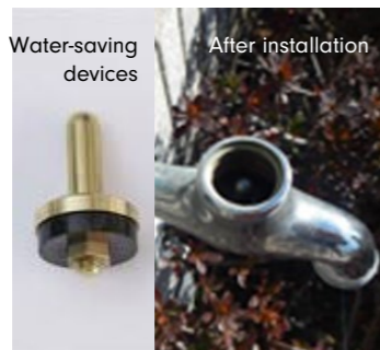
Installation of water-saving devices.
