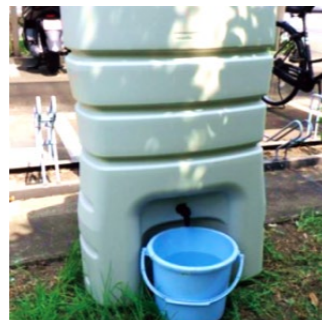
In an effort to save water, well water and rainwater are used to drain toilets as well as to water the plants in the facility.
