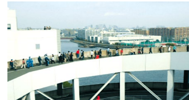
Slope supports people evacuating to the roof top
