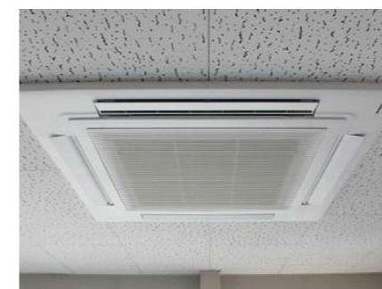
Updating air-conditioning equipment
