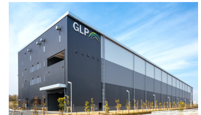
GLP Kawajima In September 2020, during the approach of Typhoon #12, the local government asked for the use of GLP Kawajima as an emergency shelter based on the disaster agreement.
