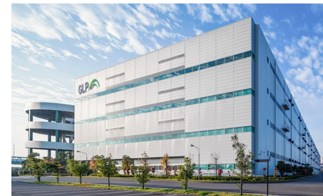
GLP Yokohama (Emergency capacity: 922 people)
