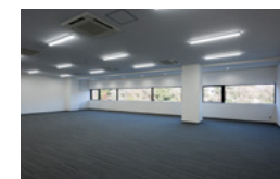
Securing Office Lighting and Power Supply
