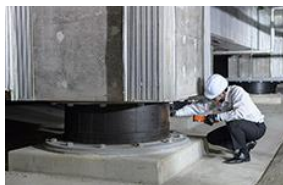
Seismic isolation structure
