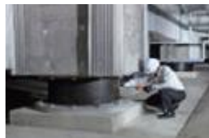
Seismic isolation structure
