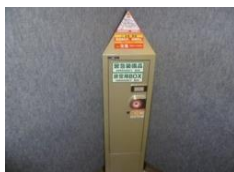
Emergency cabinet in elevators
