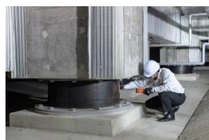
Seismic isolation structure
