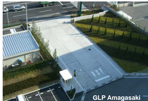
GLP Amagasaki Photocatalyst pavement (Note)
