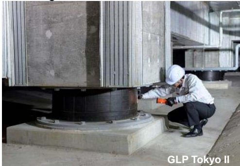
GLP Tokyo II Seismic isolation structure
